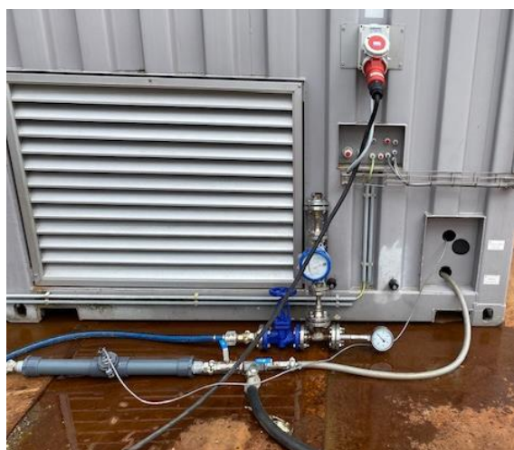
Figure 9-3: Connections to the container. The tube with the BioGeorge is situated on the outside of the container. On the floor left in the figure.
