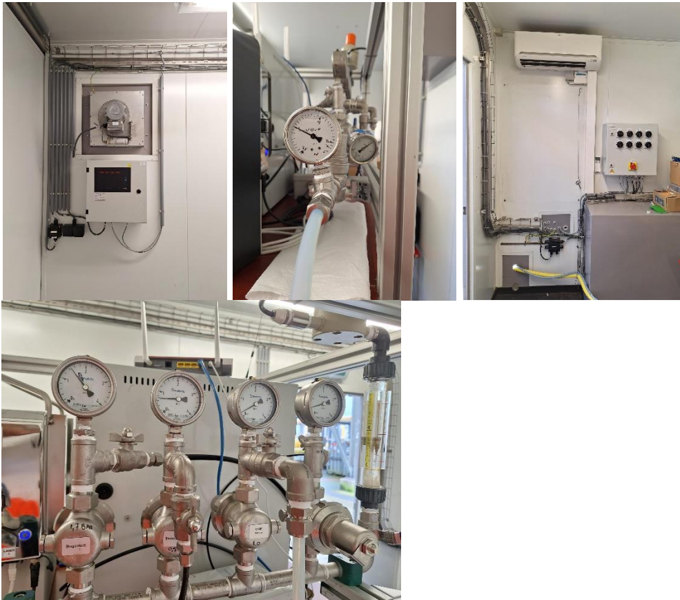
Figure 8-4: Several pictures that show the inside of the container with the pressure reduction valve (5-->2 bars) and the reduction valves for each individual sensor
