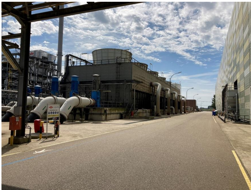
Figure 8-2: Side view of the Elsta cooling tower where the cooling water is supplied to the plants. This is the side that is on the upper side in the previous figure.
